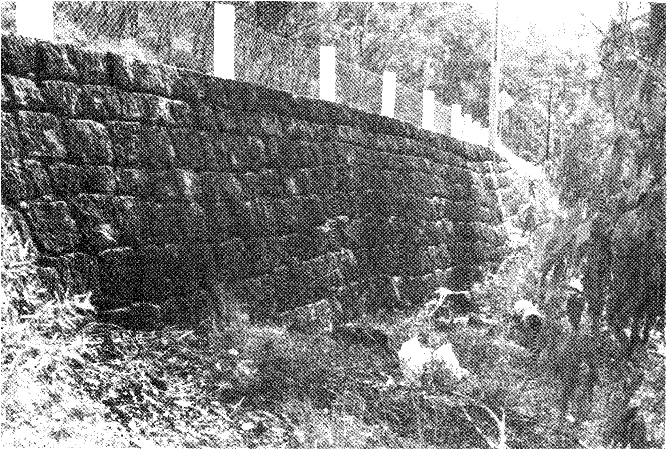
Fig. 9: Stone retaining wall on the descent to Wisemans Ferry.
