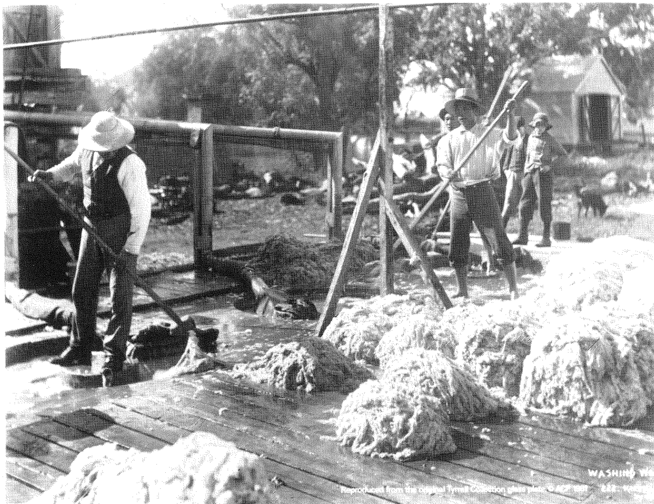
Fig. 2: This Kerry photograph, taken in the last decades of the last century, shows Chinese workers operating an unidentified woolscour. Three William's boxes can be seen in the rinsing tank, with boarded work-platforms between them. Water is supplied from elevated tanks (upper left) through pipes to slotted nozzles in each William's box. The scoured wool lies in heaps on the draining floor to the right, the hydro-extractor being perhaps to the right of the photograph. The man to the left stands on the oval 'tub' in the middle of one of the boxes, removing rinsed wool with a fork. (Reproduced with the kind permission of Australian Consolidated Press.)
