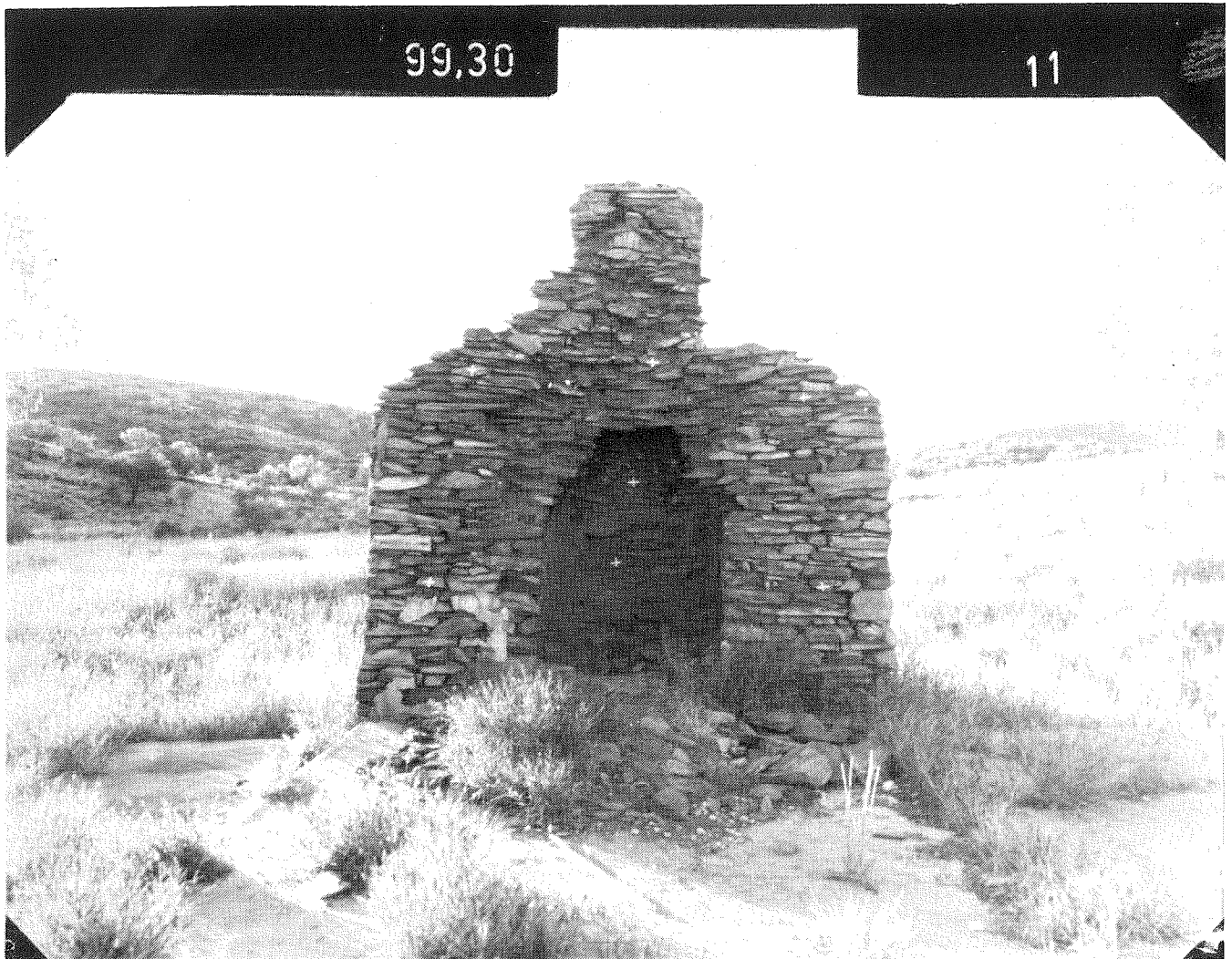
Fig. 2: Survey photograph of the Police Residence chimney taken from the right-hand base terminal. The original negative is 83\text{mm} \times 117\text{mm} . The camera calibrated focal length ( 99.30\text{mm} ), and the photograph number (11), are recorded on the photograph during exposure.
