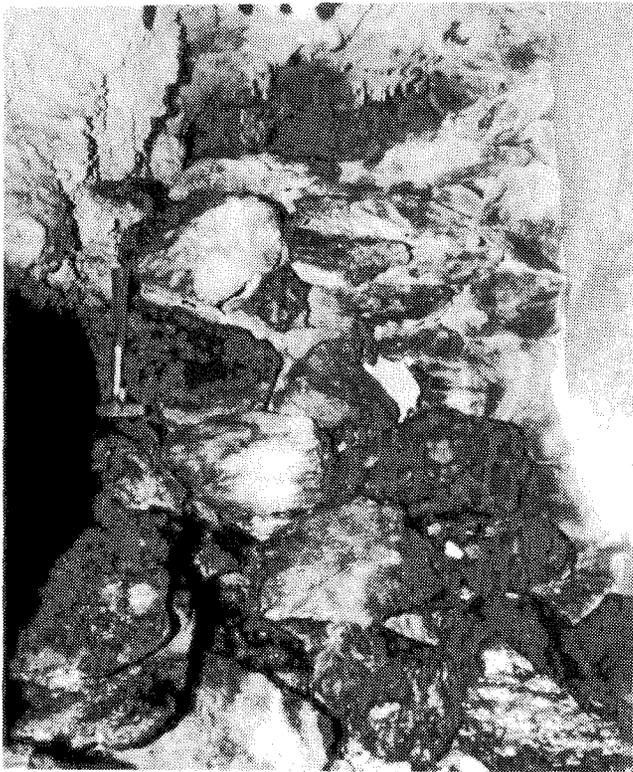
Fig. 4: Upstream wall constructed in the cave system beneath the railbed (Photo: A. McConnell)
