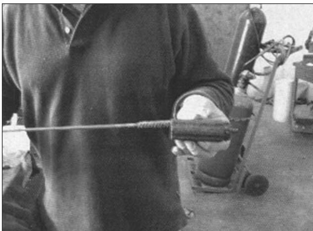
Fig. 7: Cleaning of bores with brush.
