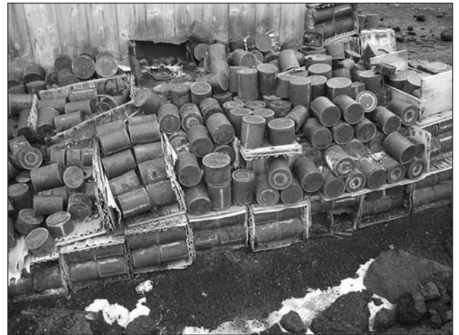
Fig. 9: Cape Royds, south side before stores removal.
