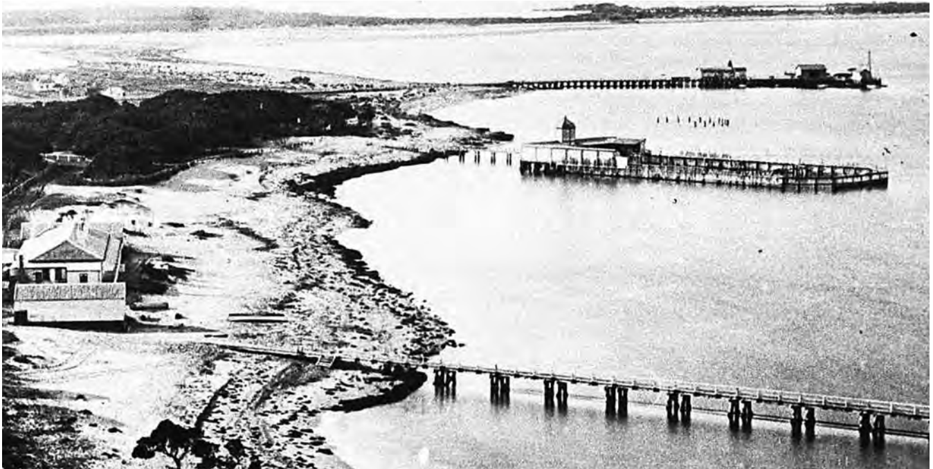
Fig. 4: Maritime infrastructure in Queenscliff Bight. Boat jetty and pilot station (foreground and left), ladies' baths (centre), remains of Queenscliff Bathing Company Baths being dismantled and Fishermens Pier (at top) c. 1882. Photo PH 292, Queenscliffe Historical Museum Collection
