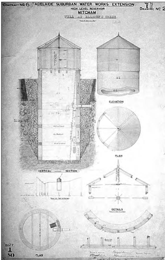
Fig. 3: The original 1879 drawings for the Mitcham High Level Reservoir well at Ellison's Creek. Contract no. 6, Drawing no. 2. 1878. Engineering and Water Supply Department n.d. (a)
