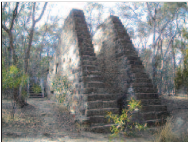
Figure 3: Stone abutments of the Garfield water wheel (P. Davies).
