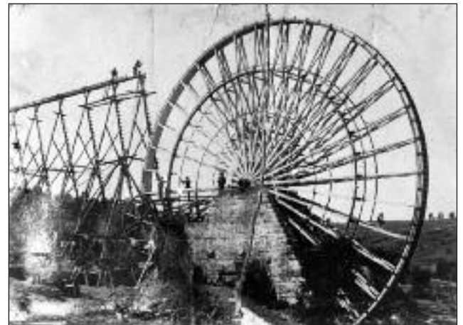
Figure 4: The Garfield water wheel under construction (State Library of Victoria image H2009.38/25).
