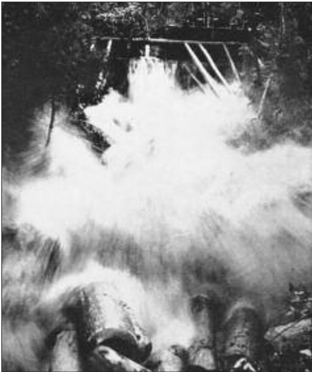
Figure 2: A dam tripped, disgorging its contents of water and kauri logs (Matakohe Kauri Museum).
