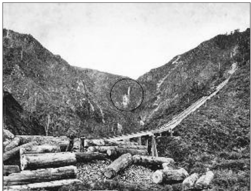
Figure 7: Billygoat Incline (maximum gradient: 1:2.3) showing empty bogeys being winched up. Billygoat Falls can be seen near the centre (circled) (DoC Kauaeranga collection).
