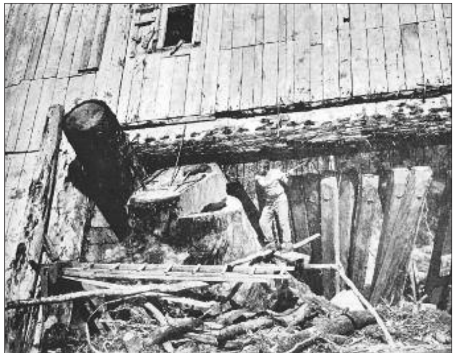
Figure 9: A stump jammed in the gate of a dam after a drive. This caused a back-up of most of the other logs in the dam (DoC Kauaeranga Collection).
