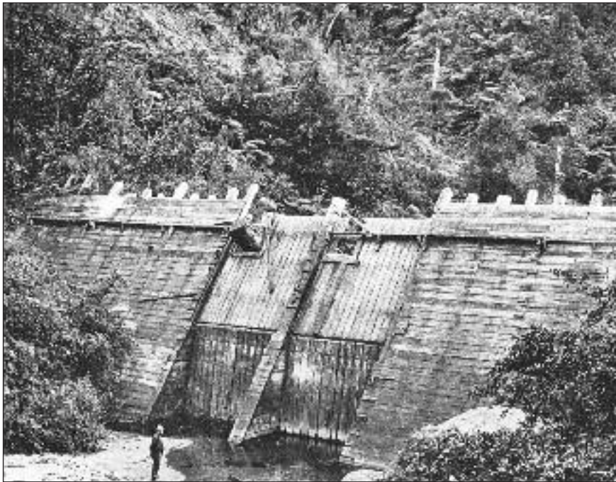
Figure 4: This large dam was on the Kapowai River, Coromandel Peninsula. The double gate was designed to let the water rush away quickly and give strength to the construction. The gates have been closed to allow the dam to refill. Over 8 million cubic metres of kauri were driven through this dam (Matakohe Kauri Museum).
